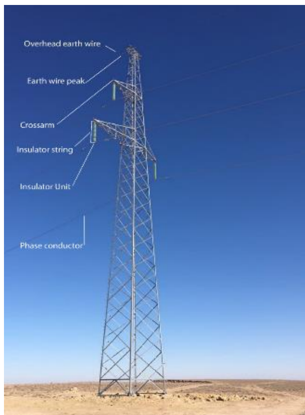
Figure 14: Components of an OHTL (source: Juru)
