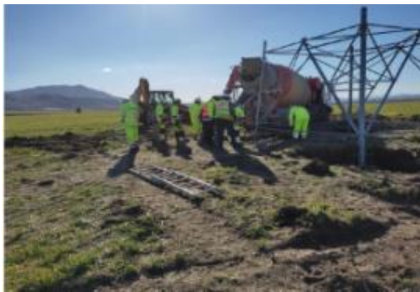
Figure 39: Example of tower assembly process (source: NJDA 2022)
