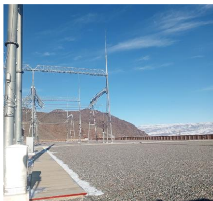
Figure 8: Spare bay for the 500 kV Kemin-Balykchy OHTL in the Kemin substation (source: Kemin Balykchy inception report, December 2024)
