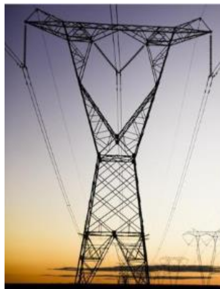
Figure 28: Self-supporting 500 kV Steel Lattice Suspension Tower (single circuit) (source: Juru)
