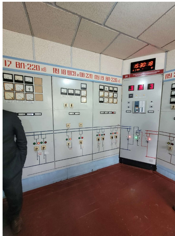
Figure 20: Old version analogue type control panel of Kristall.
