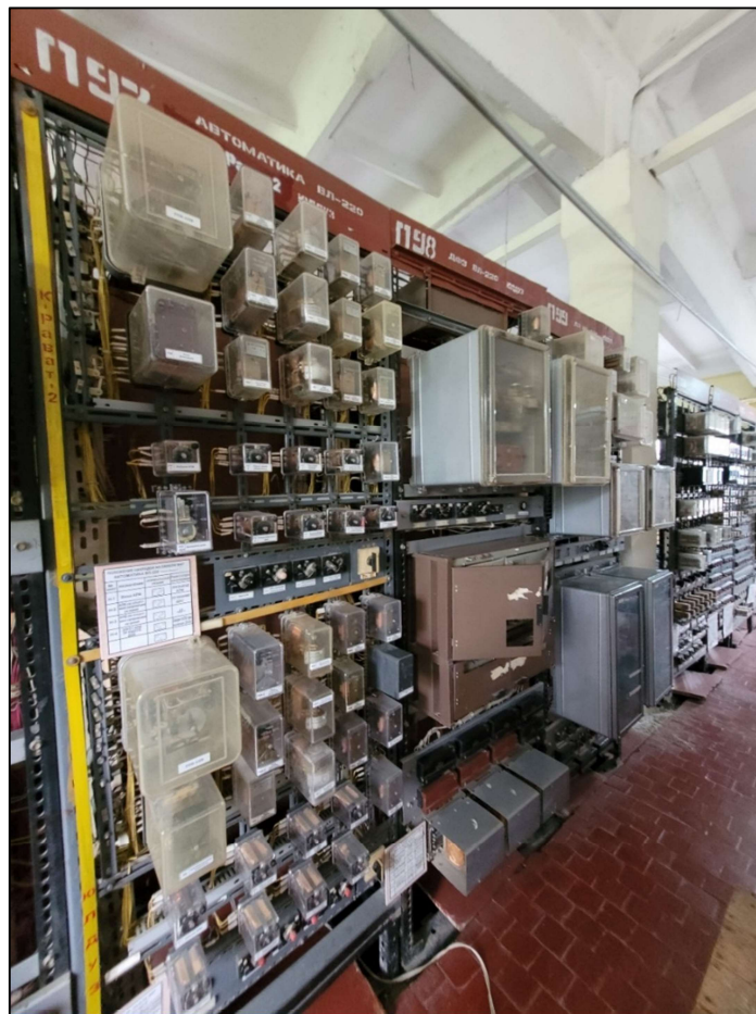
Figure 22: Current Protection System Equipment of 220 kV Yulduz Line on Kristall SS
