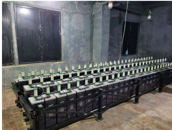
Figure 17: Battery bank of Kristall SS
