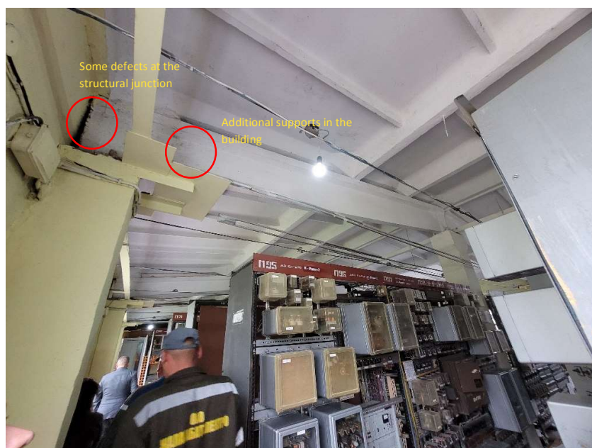
Figure 4: Part of Control & protection building with some defects.
