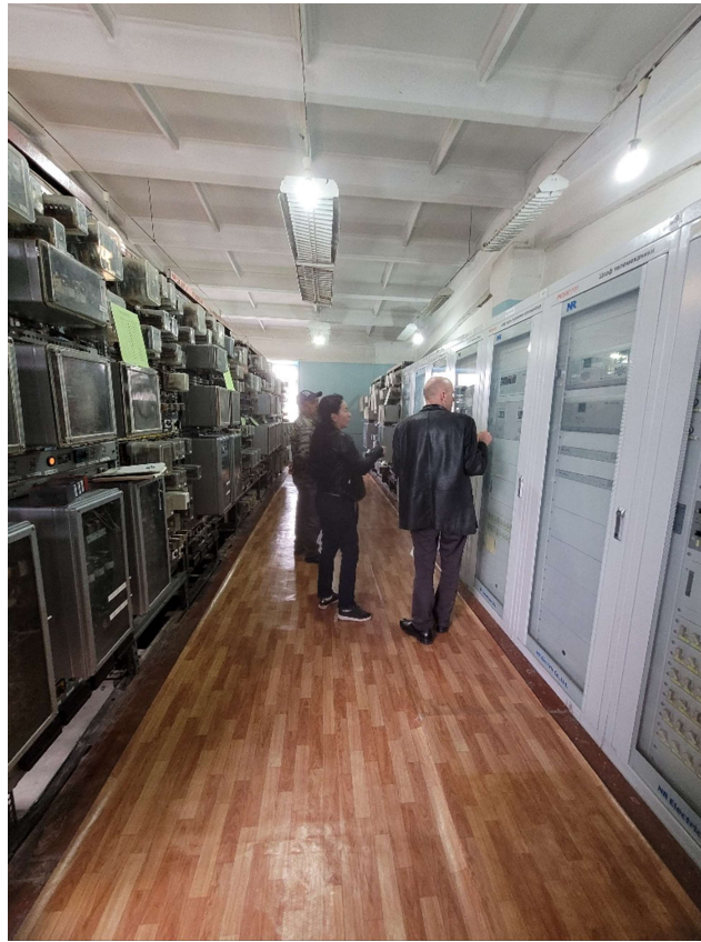
Figure 46: Electromechanics and digital (Datka 1-2) relays in Lochin substation.
