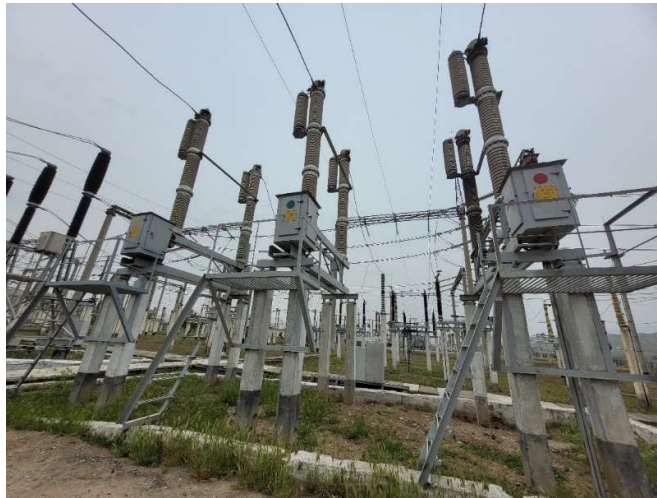
Figure 14: Old circuit breaker at autotransformer feeder, oil filled type and oil leaks exist.
