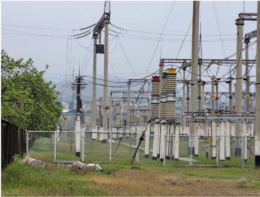
Figure 6: Vegetation beneath switchgear and misalignment of poles.
