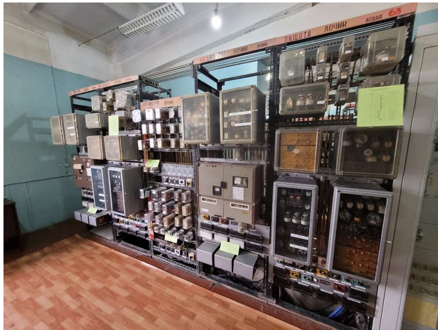
Figure 47: Lochin line (left-right) differential & distance protection.
