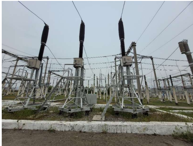
Figure 13: Circuit breakers in Kristall in good condition and relatively new.
