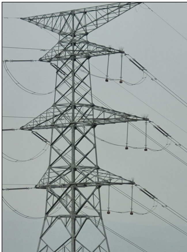
Figure 41: Bird Guard Application Example from A 110-Kv Tower in Finland 7 .
