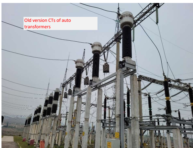
Figure 12: Old CTs of autotransformer.
