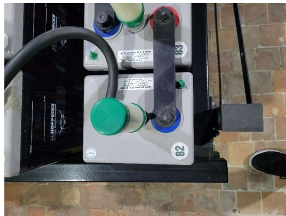
Figure 18: Kristall SS batteries, with V L 2-550 model with liquid electrolyte (lead acid, dilute sulfuric acid).
