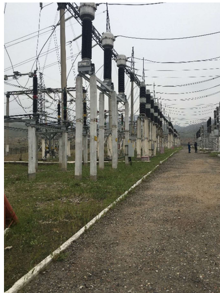
Figure 7: Vegetation beneath switchgear, non-planar ground in the entire switchgear.
