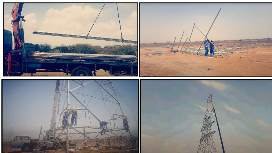
Figure 43: Some Stages of a Tower Erection Process
