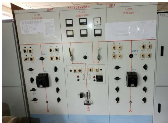
Figure 19: Battery charger system with redundant equipment.
