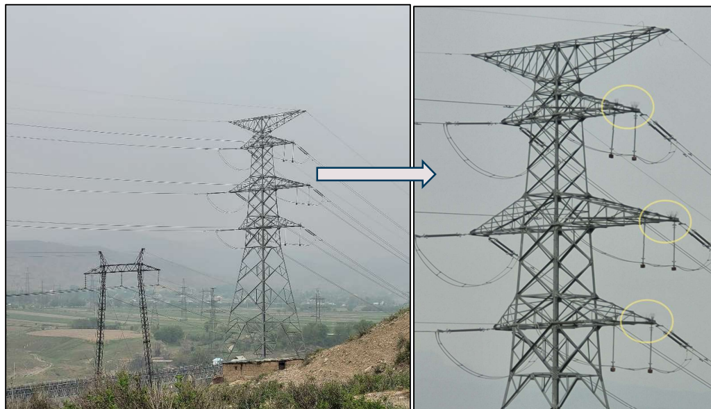
Figure 42: A Tower of Kristall-Datka Line with Bird Guards Near the Kristall SS
