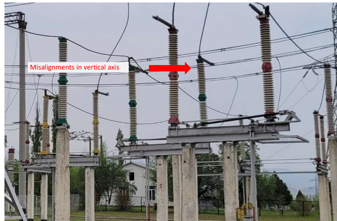
Figure 15: Disconnectors in Kristall SS in a poor condition.
