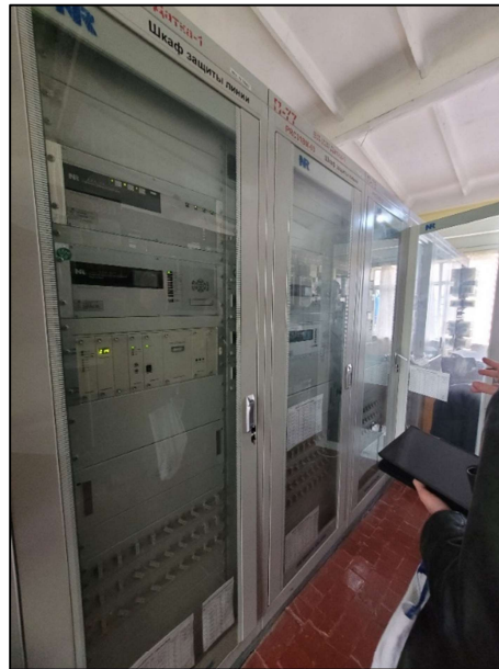
Figure 23: Digital Relay Line Protection Cabinets of Datka Lines on the Kristall SS
