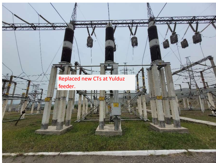
Figure 11: Replaced new CTs
