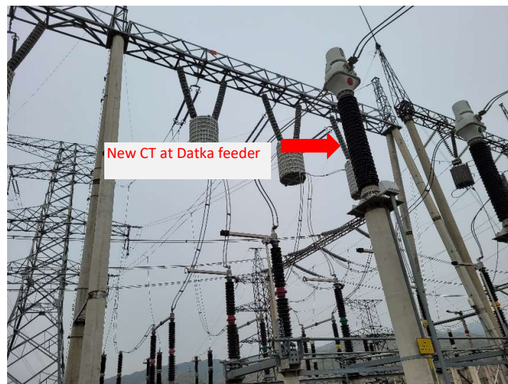
Figure 10: CTs of Datka feeder
